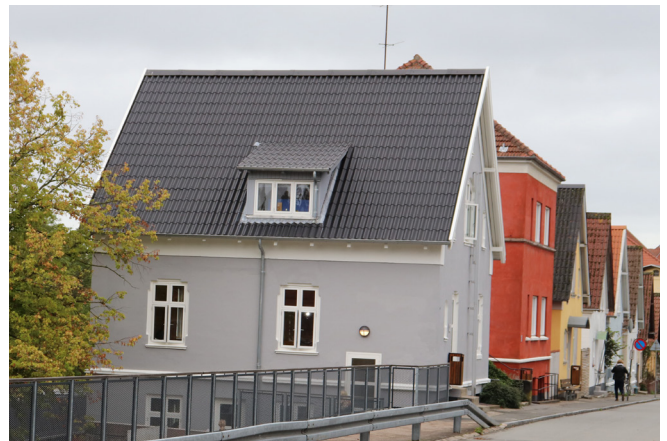
The first villa on the road, where the 5th grade is located on the top floor, previously had really stale air and a high CO 2 level.
